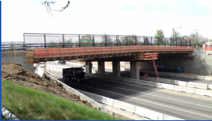
Knox Court bridge
